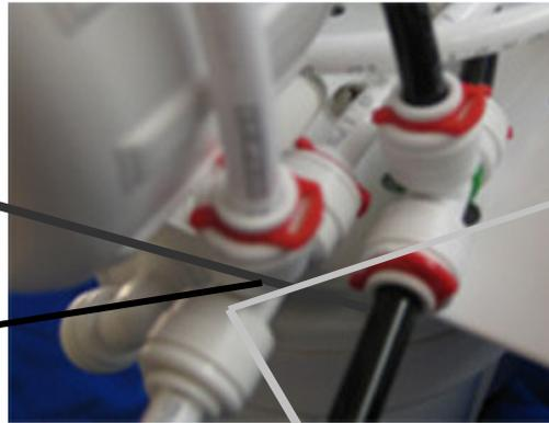
White tubing connects to tank from TEE PIECE. One line brings water to and from tank.
